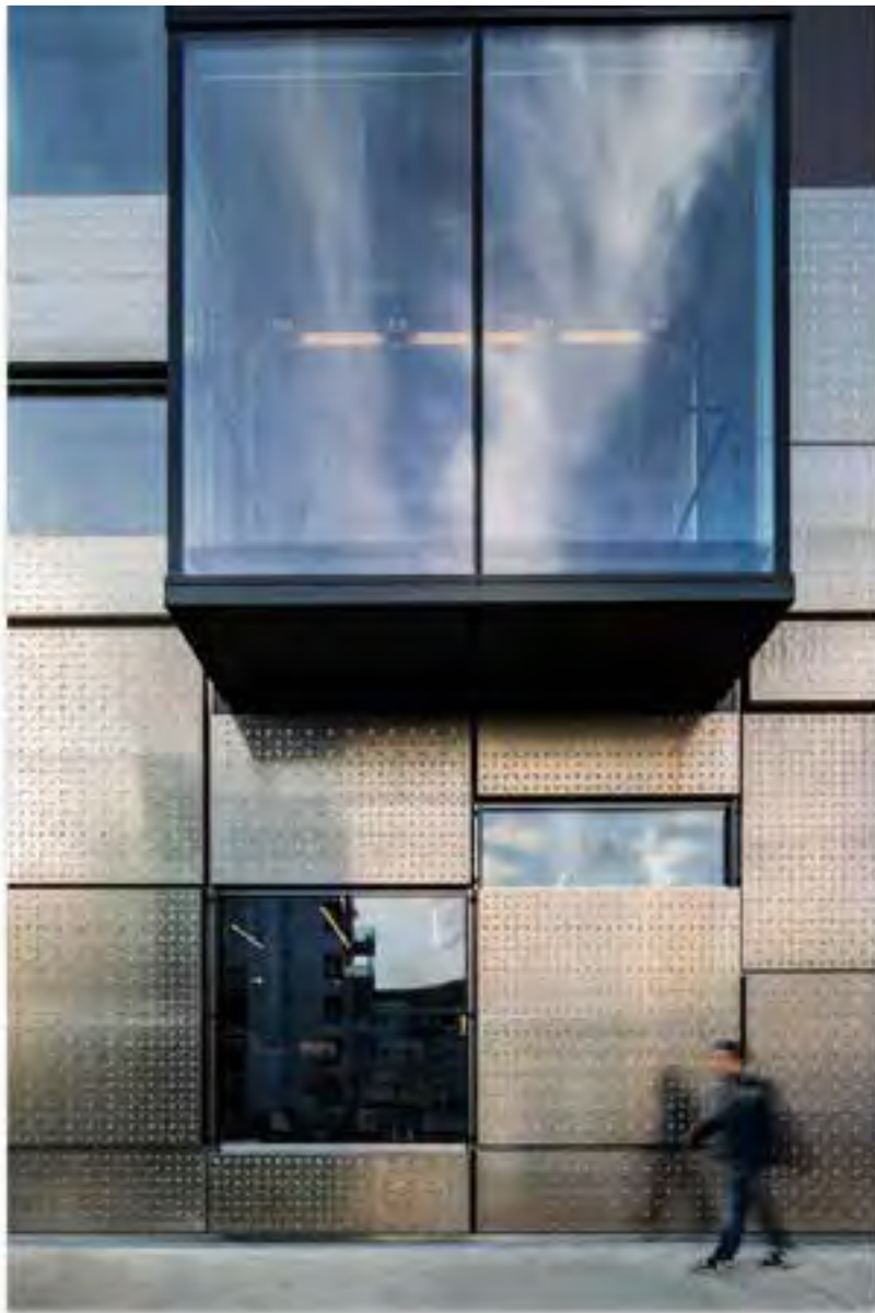
The studio used pre-fabricated raw aluminum elements that clad the building's exterior compose a palette of depth, breadth and length. 300 square millimeter square aluminum elements are protruding from the wall at varying distances, only pierced by large cantilevered box-shaped windows punctuating the rhythm of the aluminum surface. The metal cassette shifts according to the weather conditions of the west coast and reinforces the metallic effect of the aluminum.
