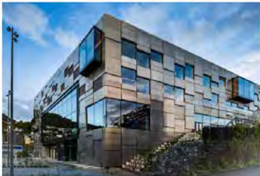
900 seawater-durable crude aluminum elements protrude from the wall at varying distances
