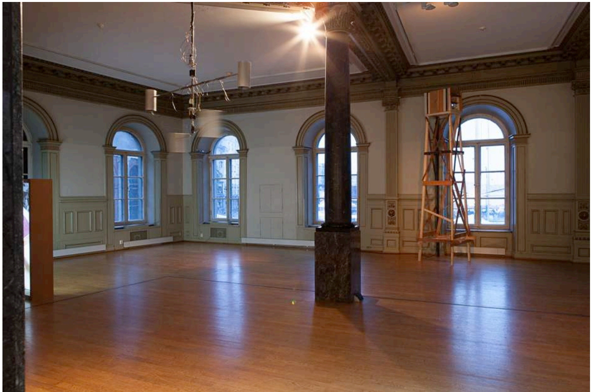
Figure 65, The frame seen from the door.
