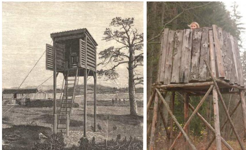
Figure 26, (Left) In 1838–39 a temporary research station was erected in Bossekop in order to study Aurora Borealis and earth magnetism. This is the weather hut. Figure 27, (Right) Observational tower for hunting.
