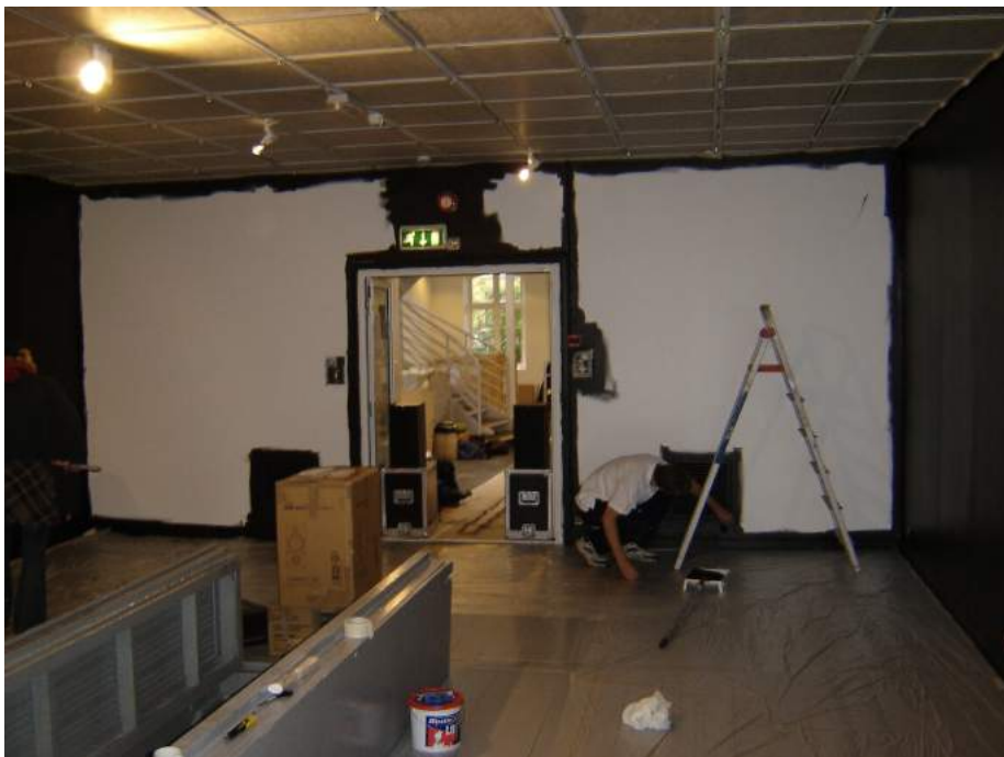
Figure 3.24: The installation was prepared in five hectic days and nights.
